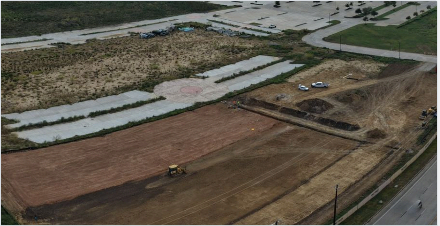
FIG. 03 Retail 3 fine-graded pad (left) and trench runs with site trailers at the west end, 2026-10-06.
