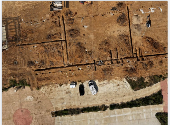
FIG. 07 Retail 5 footing excavations and spoil.
