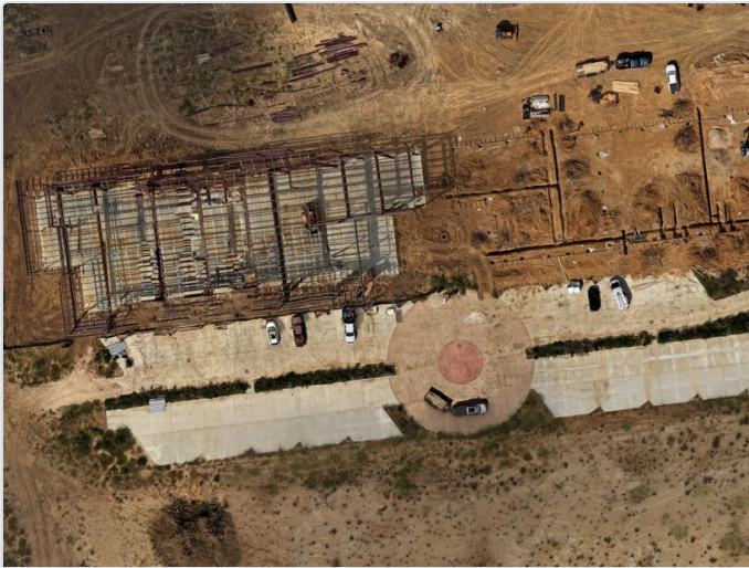
FIG. 06 Retail 4 steel frame and slab.
